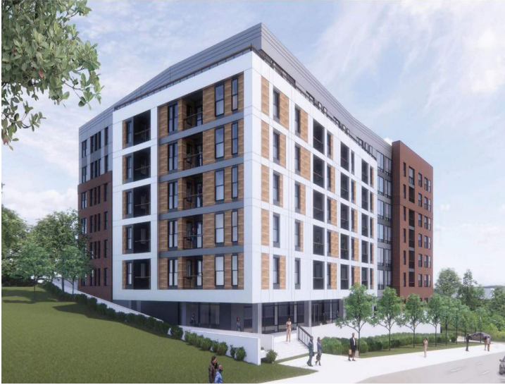
Southwest Corner from Central Ave
